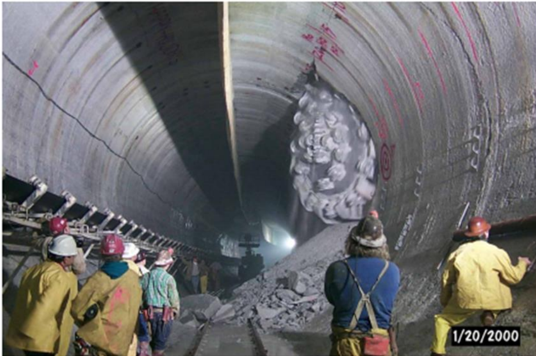
Figure 5-1. Full-profile machine (Robbins TBM) excavating a tunnel in Chicago, IL, USA. The cutter heads seen in the picture have broken through to the main tunnel created with the TBM method. Source: Lach et al. 2000
