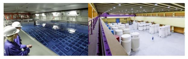
Photo 8. Wet storage of nuclear waste in Sweden (Source IAEA). Photo 9. Dry storage in Switzerland (Source Zwilag)
